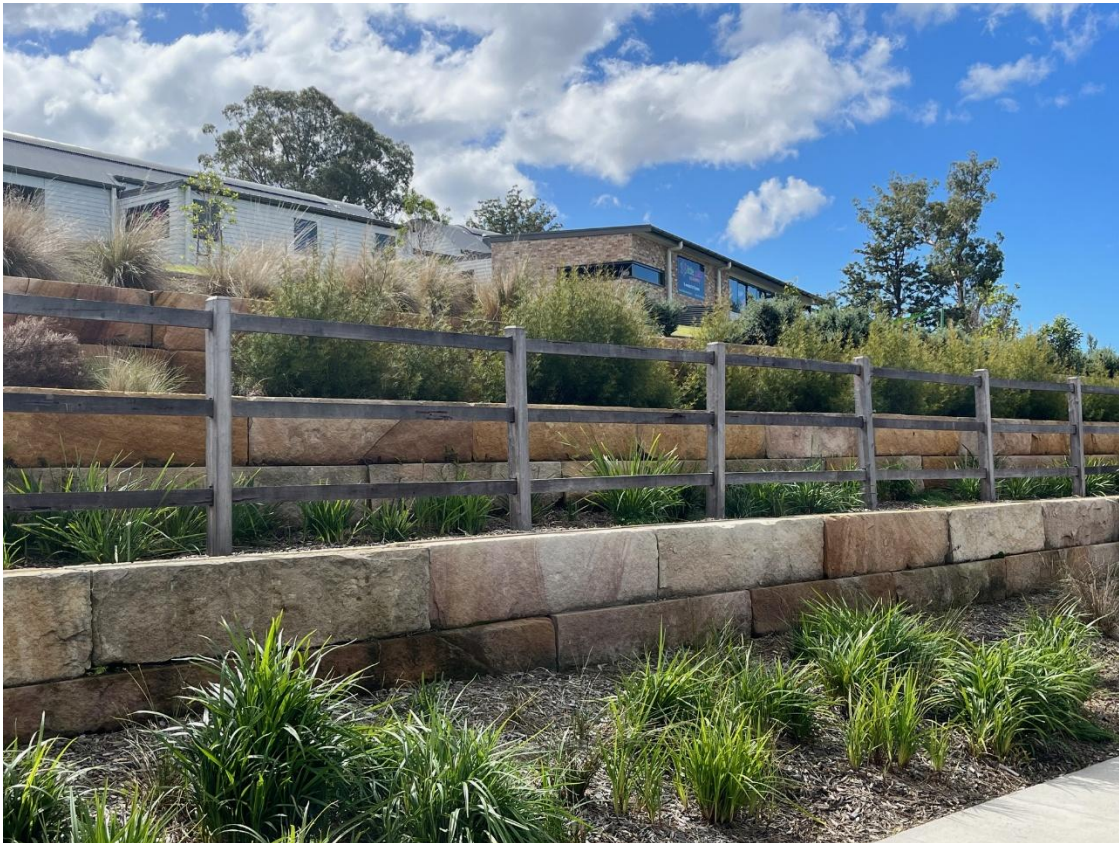
Figure 7: Example of 2m tiered sandstone retaining wall in Wongawilli estate in Wollongong
